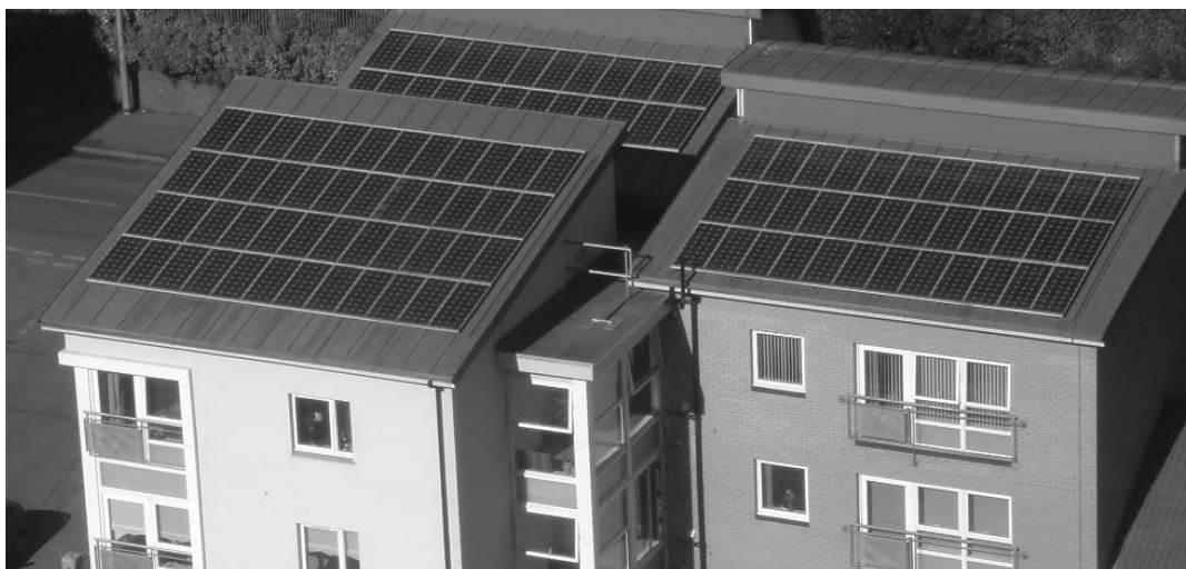
Some 70 polycrystalline photovoltaic solar panels, made by Sharp and covering 66 square meters, on homes owned by the Queen’s Cross Housing Association, Panmure Street, Glasgow, Scotland. Unfortunately, they only generate about 8.75 kilowatts—enough to power 87 100w lightbulbs. Photo courtesy Currys.
